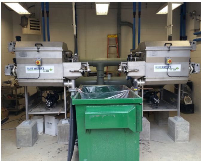
Blue Water's Eco MAT™ installed in Valparaiso, IN.
