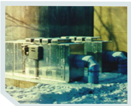
Aluminum Outside Chlorine Scrubber - 150 lb Capacity
