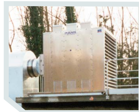
Aluminum Outside Chlorine Scrubber - 150 lb Capacity
