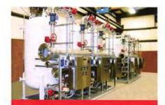
High efficiency upflow regenerated Packed Bed nitrate removal systems minimize waste and
