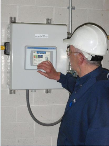
**Description:** The PHi-300 series mixer is unique in that it utilizes large air bubbles which are sequentially injected in a liquid to create powerful mixing currents. The system is contained in an 18"x16"x81/2" NEMA-4X enclosure and consists of three major components:
