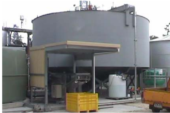
Clarifier underflow pumped directly to a V-FOLD filter
