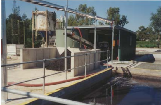
Settled winery sludge pumped to a “Day Tank” then to a V-FOLD filter
