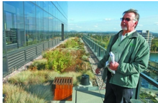
JONATHAN HOUSE / PAMPLIN MEDIA GROUP OHSU Wellness Center building engineer Mark Schnackenberg stands on a balcony that features a garden watered by the building's gray water. Central City Concern hopes to see gray water used at a 16-story high-rise apartment building in Northwest Portland.
